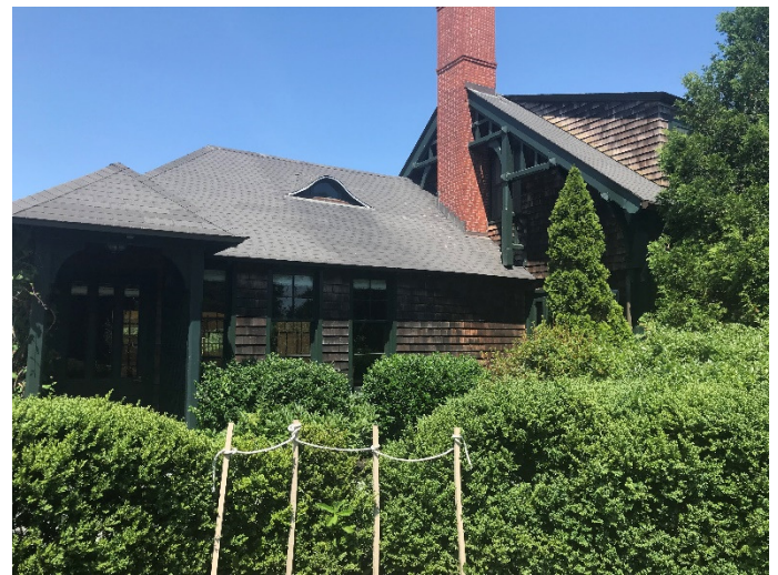
Figure 4. Present-day exterior of the Newport Marine Zoological Laboratory in Newport (photo by the author).
