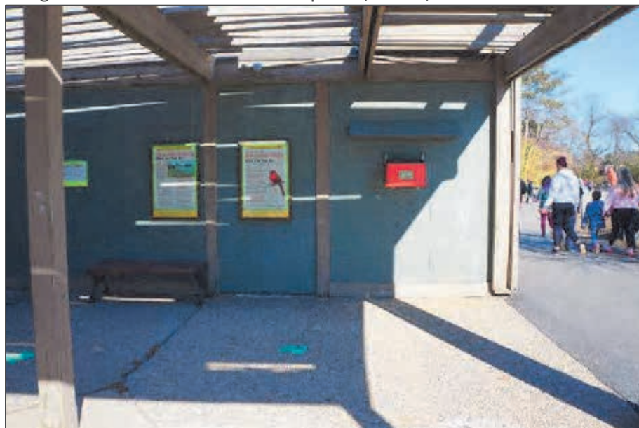
Figure 3: Rear wall of exhibit with panels, bench, and obsolete elements
