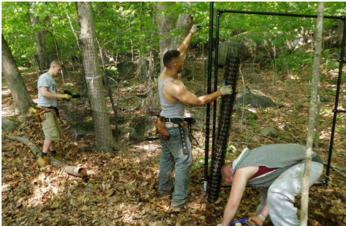
Installation of deer fencing by FHWP contractors
